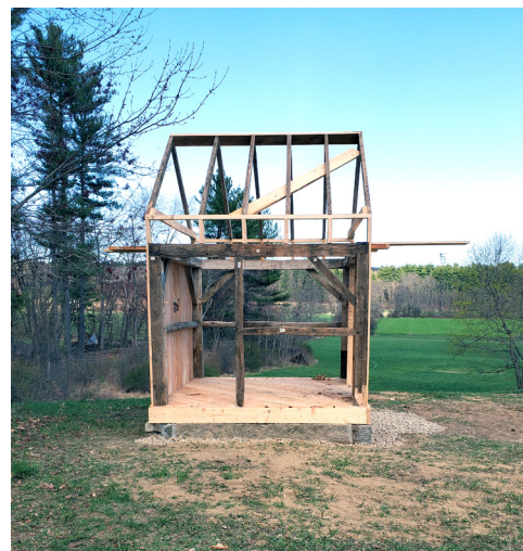
Benjamin Rideout Chicken House/Shop Being Rebuilt
