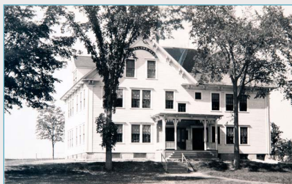
Farley Building (1921) - Second Addition
