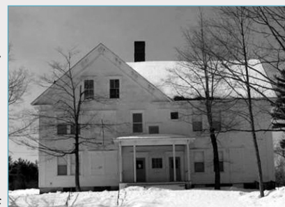
Farley Building - Today
